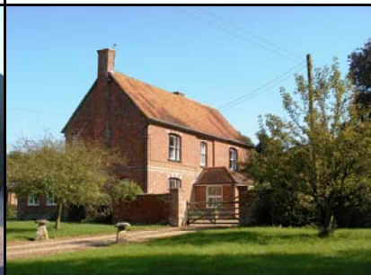
Large brick farmhouses- many of 19 th century origin.
